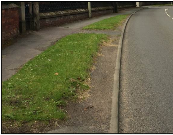
Photo 5 – A488 Hanwood o/s Church showing verge deterioration.
