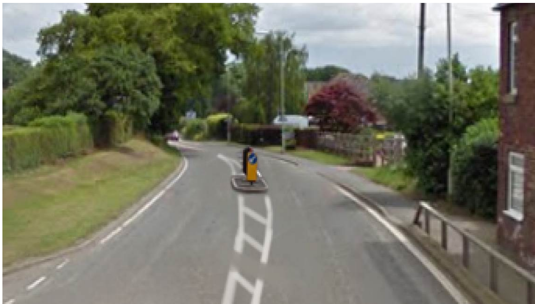
Photo 17 – A488 Hanwood east of Caradoc View showing photo impression of traffic island as a gateway feature (Option 6.3). Photo shows eastbound view - gateway signs placed in the verge would accompany the island, facing westbound traffic.
