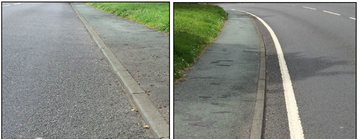
Photo's 6 and 7 – A488 Hanwood showing examples of low kerb upstand.
